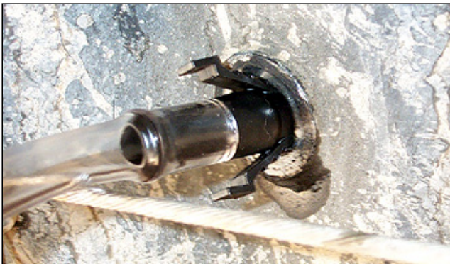
Insert the barbed end into the fill hole
